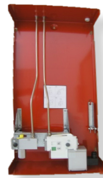
Photo 6. AK box for a "B" type damper.
